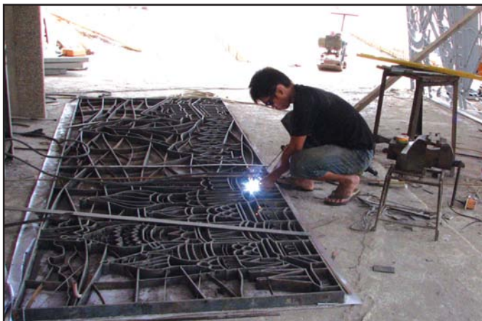
A welder works to complete the artistically-made security grills in time for the inauguration.
